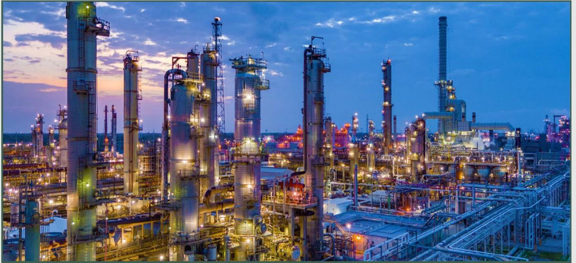
Across from—Marathon Refinery
